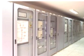
LV CONTROL AND PROTECTION PANELS
