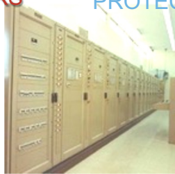
LV CONTROL AND PROTECTION PANELS
